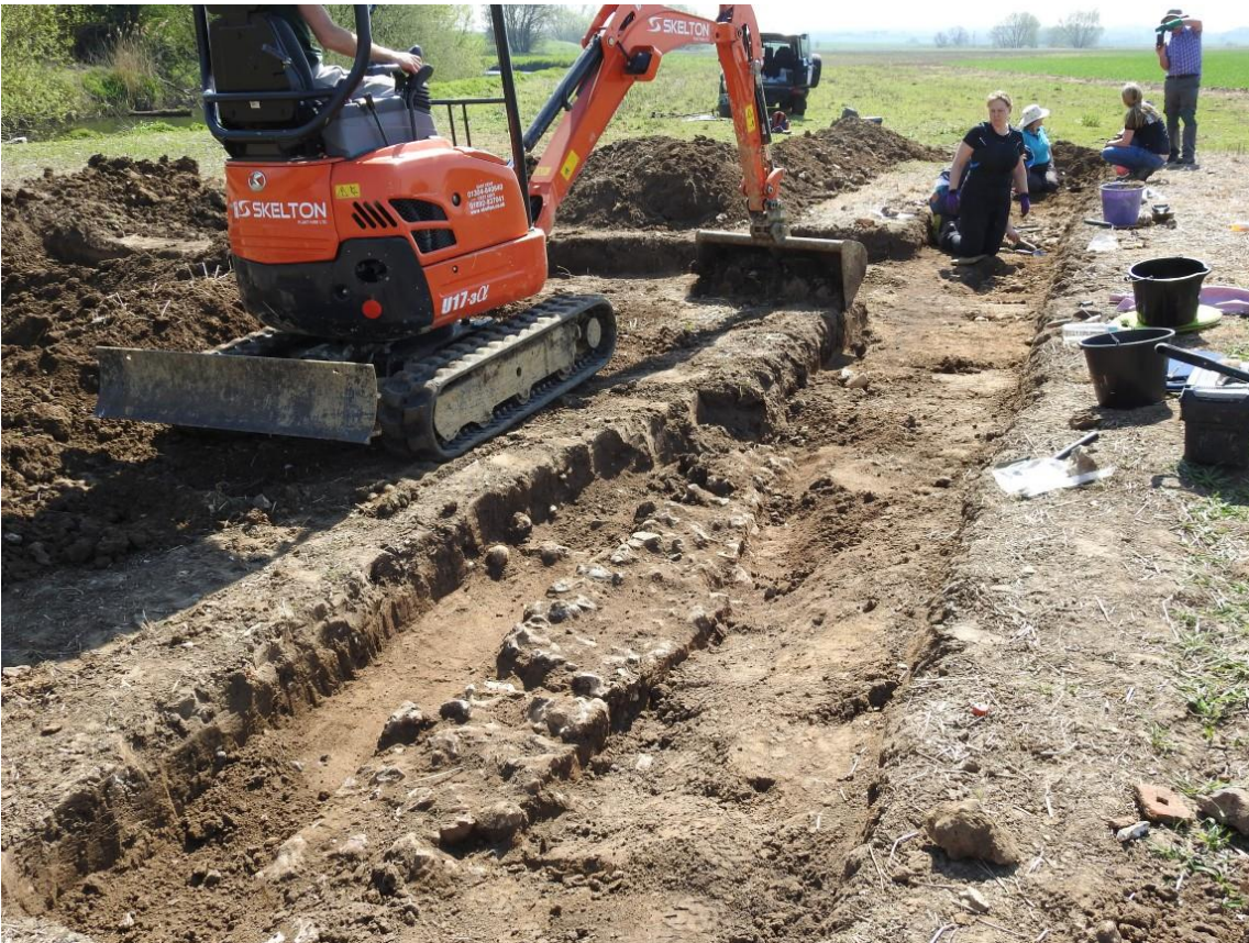
Plate 7. Removal of topsoil under archaeological supervision (Looking South)
